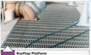
United Interlock grating offered a convenient way to construct a walkway which avoids the existing piping structures.
