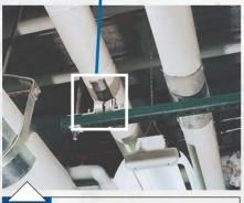
Steam Lines On Pipe Rollers Rollers on Unistrut channel keep large pipes in place while allowing for pipe expansion and contraction as temperatures change.
