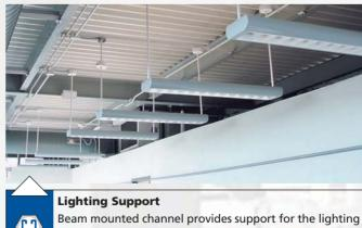
Beam mounted channel provides support for the lighting system as well as, an electrical raceway for the fixtures.
