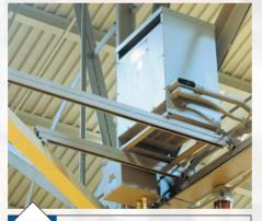
Overhead Rectifier Support Prefabricated back-to-back Unistrut sections provide plenty of beam strength for this heavy overhead rectifier.
