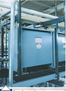
**Transformer Mounts** Extra size and weight are no problem for Unistrut Metal Framing. These equipment boxes were mounted quickly and easily without welding, drilling or special tools.
