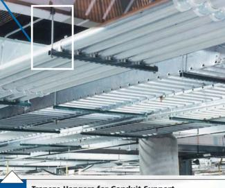
**Trapeze Hangers for Conduit Support** Trapeze hangers made from Unistrut channel suspended from the structural steel beams with Unistrut beam clamps provide dependable support for the conduit runs.
