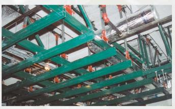
creating a clean, unobtrusive look consistent with today's equipment room aesthetics. Medical supports designed from Unistrut Metal framing have many advantages over conventional supporting methods including adjustability, mechanical connections, adaptability, and fast and efficient installation.
