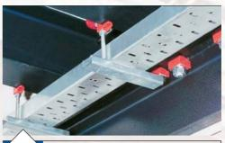
Beam-Mounted Cable Tray Supports Cable tray is supported on a Unistrut trapeze-style hanger suspended from beam clamps.
