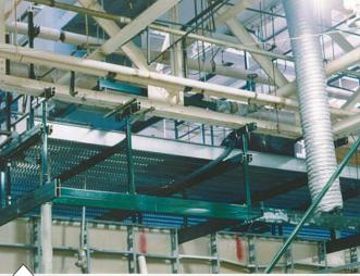
**Overhead Platform Support** Channel sections with high load bearing capabilities make the Unistrut Metal Framing System ideally suited to heavy-duty applications like the supporting structure for this overhead platform.
